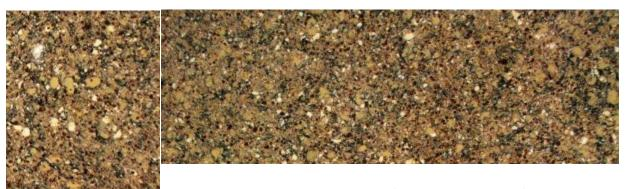
As you can see in the above example (seam shown in white), the pattern variation would have been greater if the other end of the longer piece had been used at the seam. More care and attention in the lay-out process will help to minimize potential objections by the customer.
